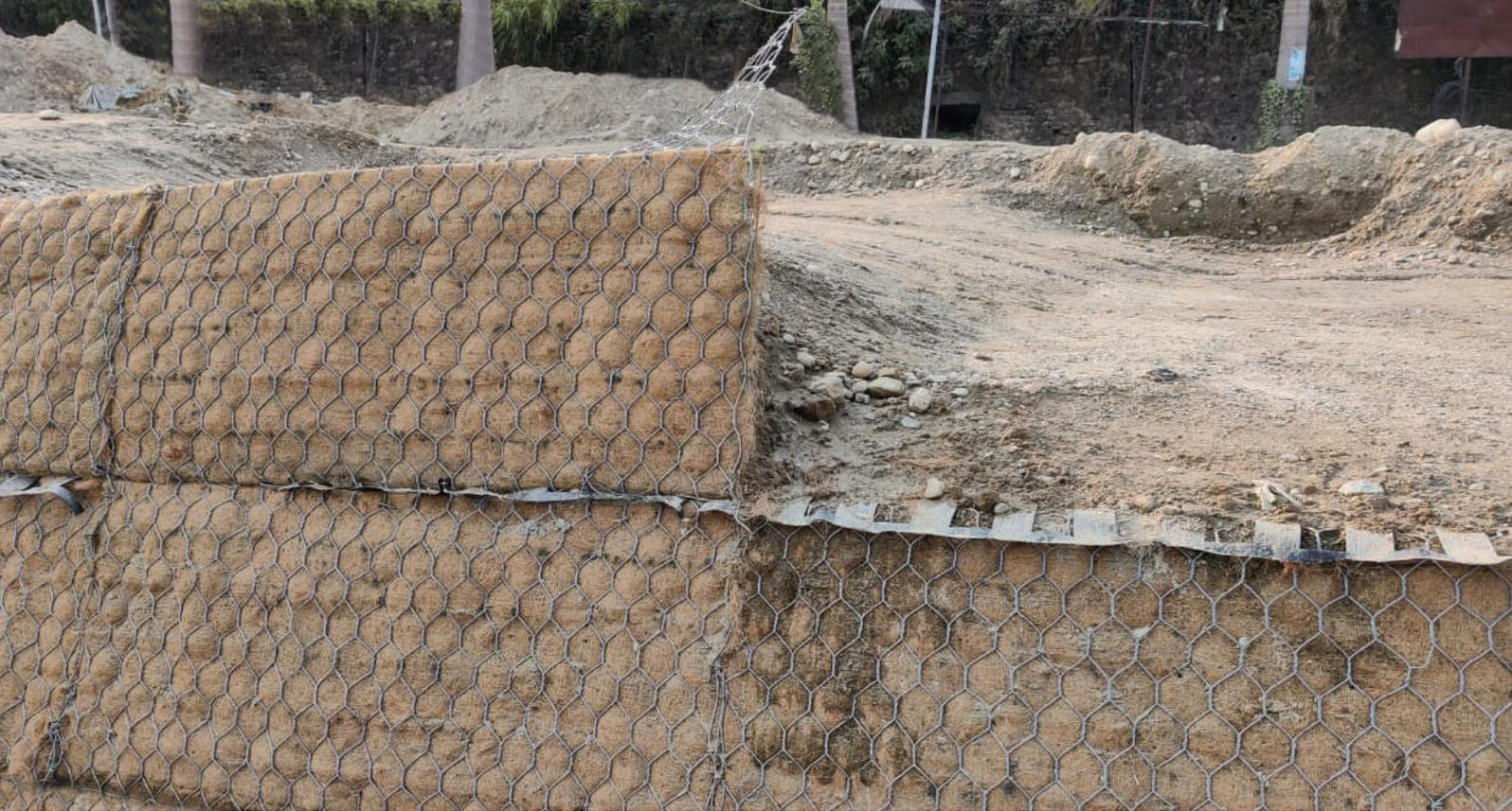
In high RSWs, a 'Green' Tailmesh sloped wall is used on top of a vertical Gabion Fascia RSW to provide a stable structure. Below is an illustrative design showing typical details of a 'Green' Tailmesh Gabion Sloping Fascia RSW.
