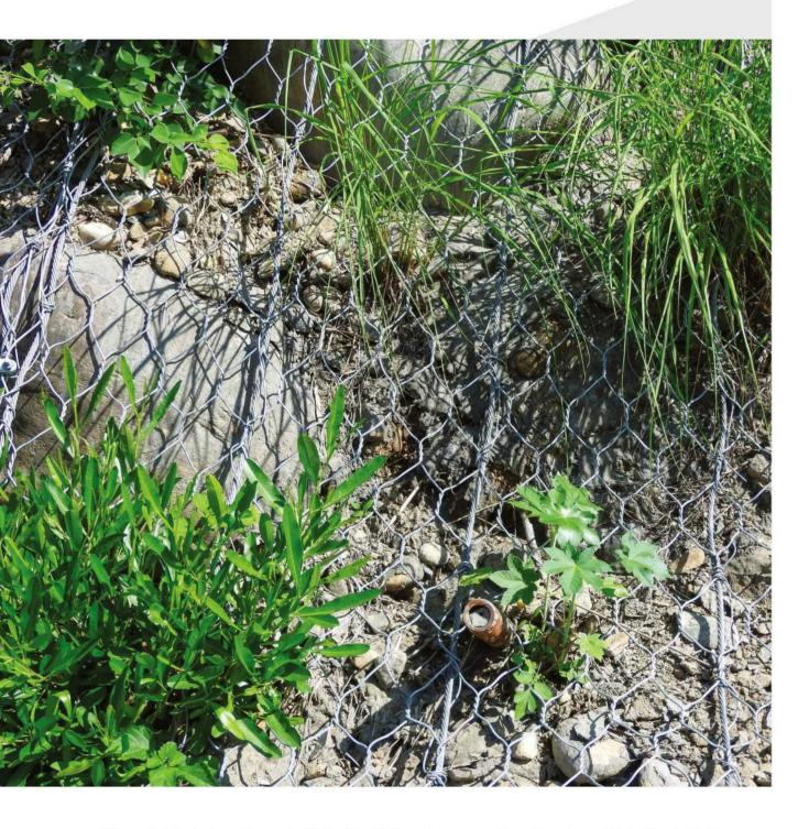
StrongNet is designed to work efficiently with its anchorage system. The stress distribution is highly even and avoids grossly heterogenous deformation in the mesh. The longitudinal wire ropes provide the strength to prevent shrinkage of the mesh under self-weight during installation and under weight of debris collected behind the mesh during its service life.
